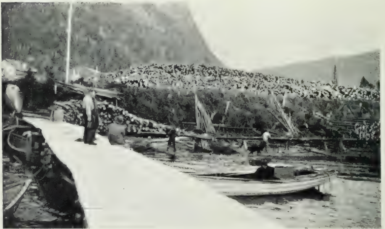
FIG. 102. STACKED SAWN PIT WOOD, CRIB PIER AND MOTOR TOWING BOAT: NEWFOUNDLAND.
